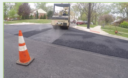
New asphalt is placed and compacted
